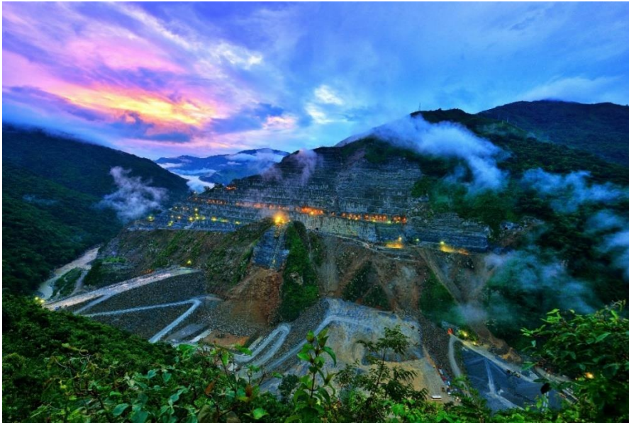
External Civil Works
