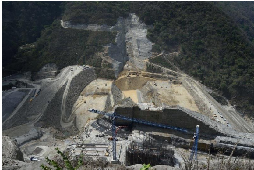
External Civil Works
